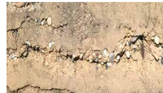
A Eroded Concrete Monument
