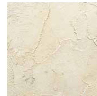
B Plaster Wall
